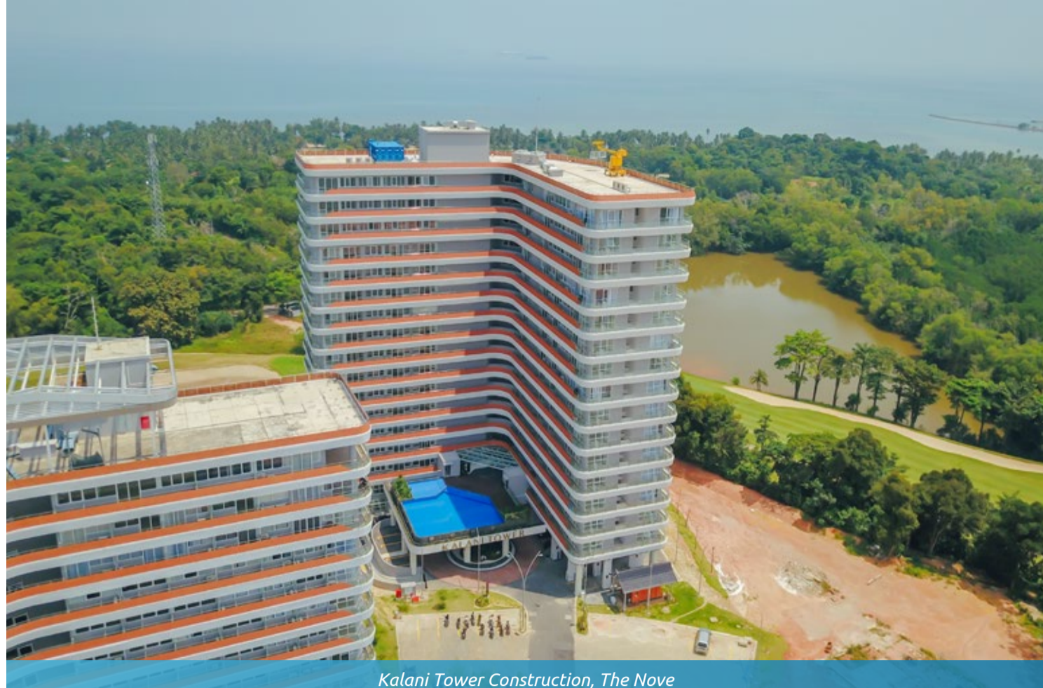
Kalani Tower Construction, The Nove
