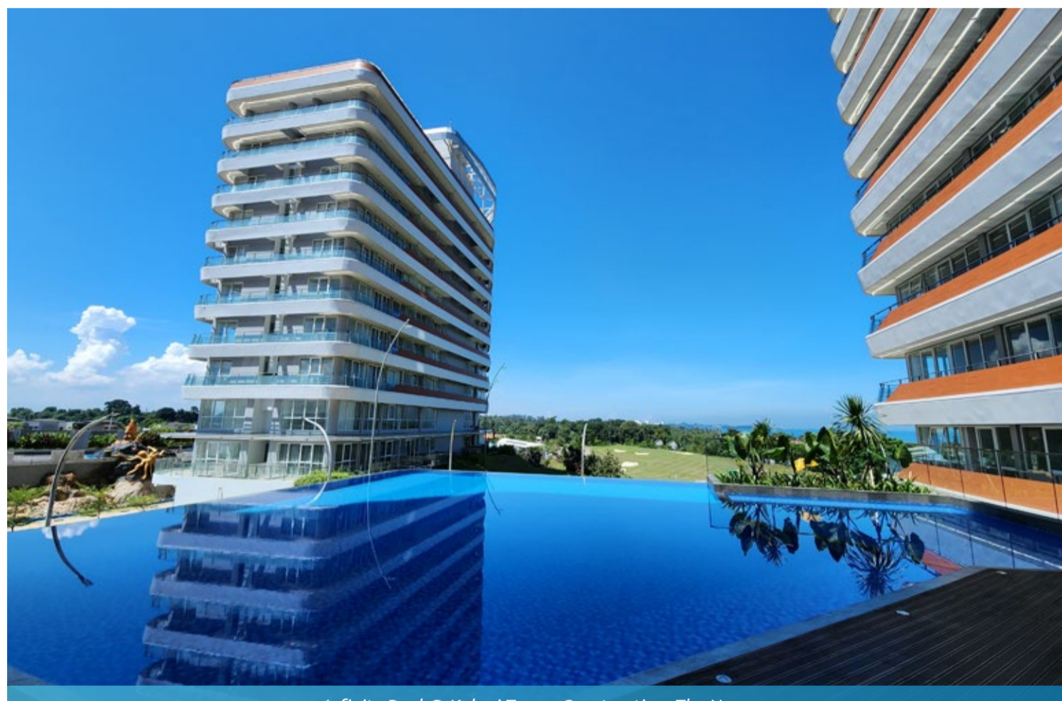
Infinity Pool @ Kalani Tower Construction, The Nove
