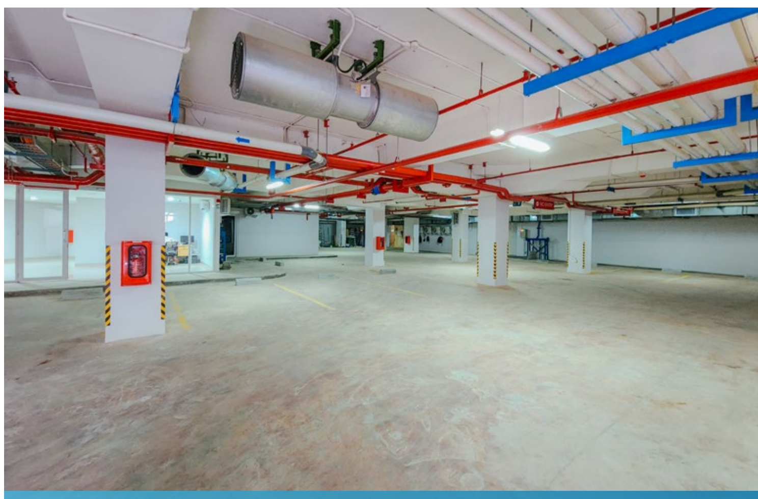
Basement Parking @ Kalani Tower
