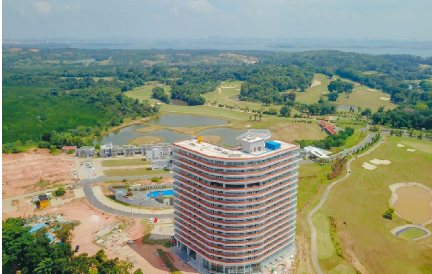
Kalani Tower Construction, The Nove
