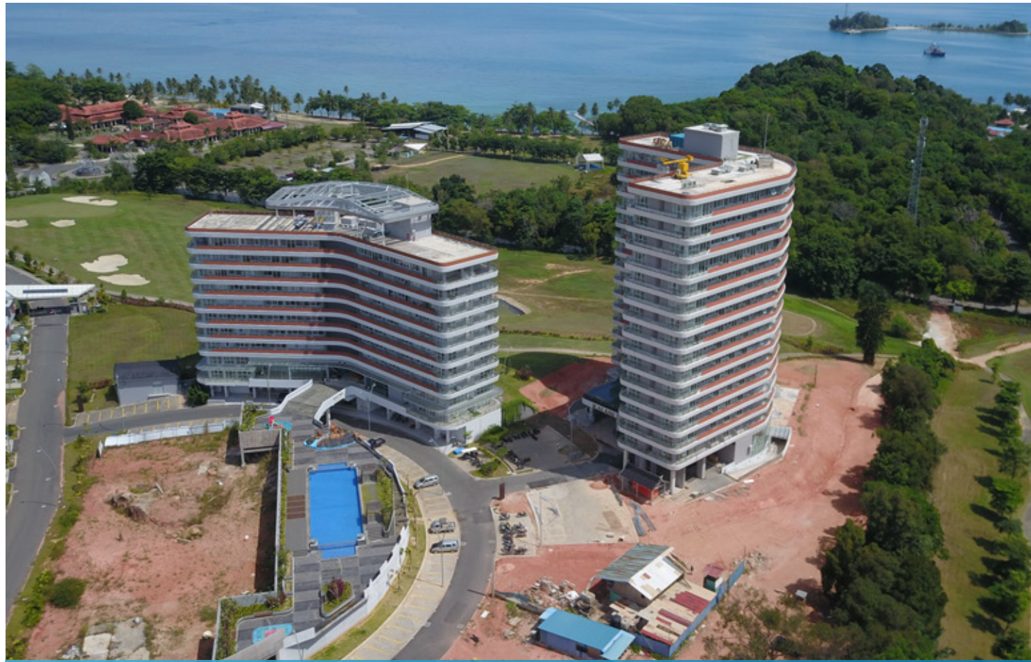
Kalani Tower Construction, The Nove
