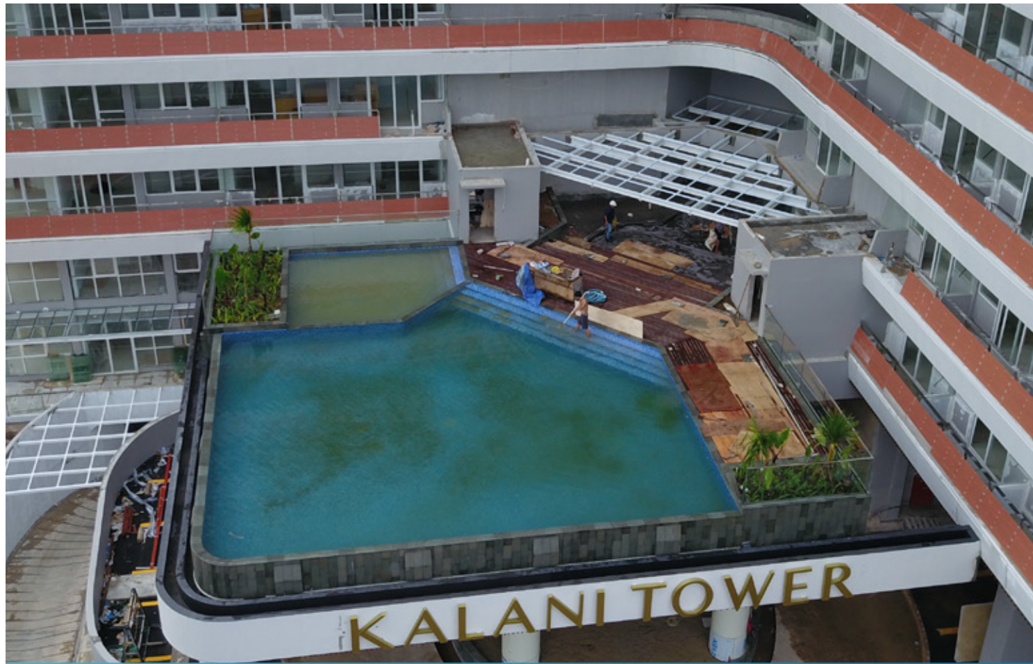
Infinity Pool @ Kalani Tower Construction, The Nove
