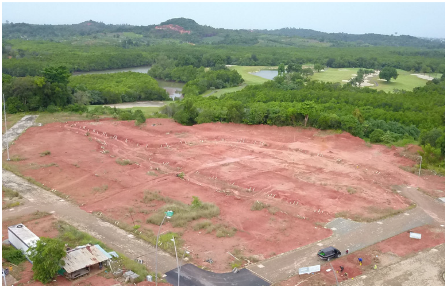
Construction of Landed House phase 2
