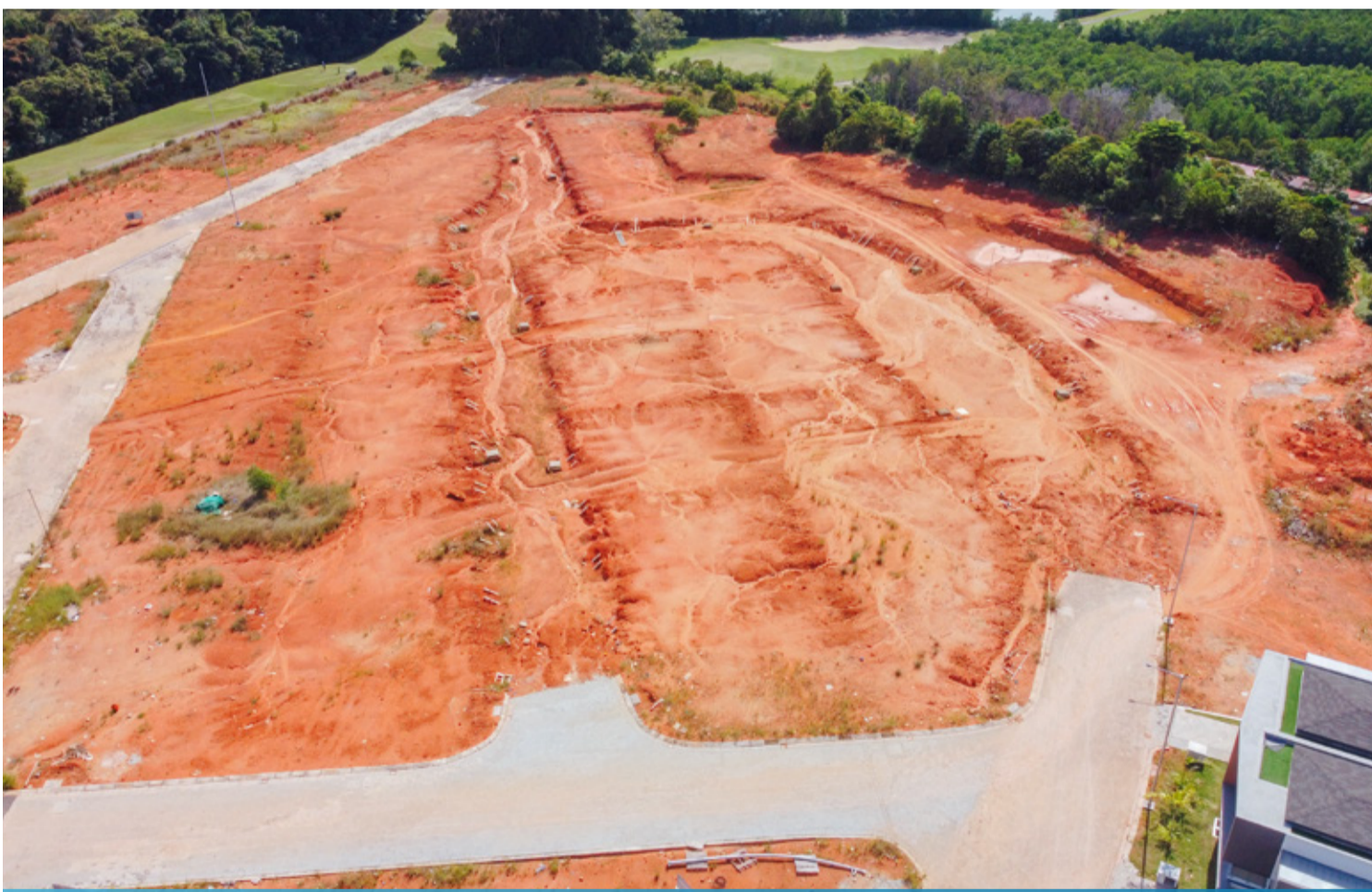
Construction of Landed House phase 2
