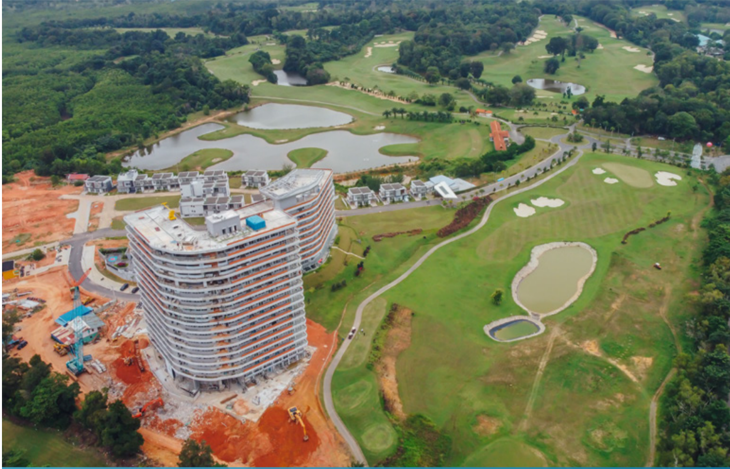
Kalani Tower Construction, The Nove
