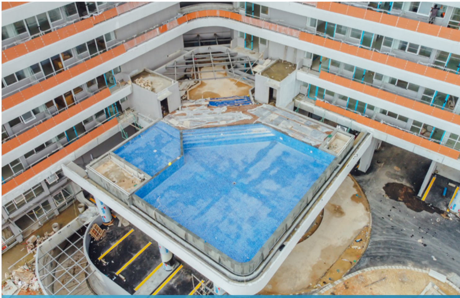
Infinity Pool @ Kalani Tower Construction, The Nove
